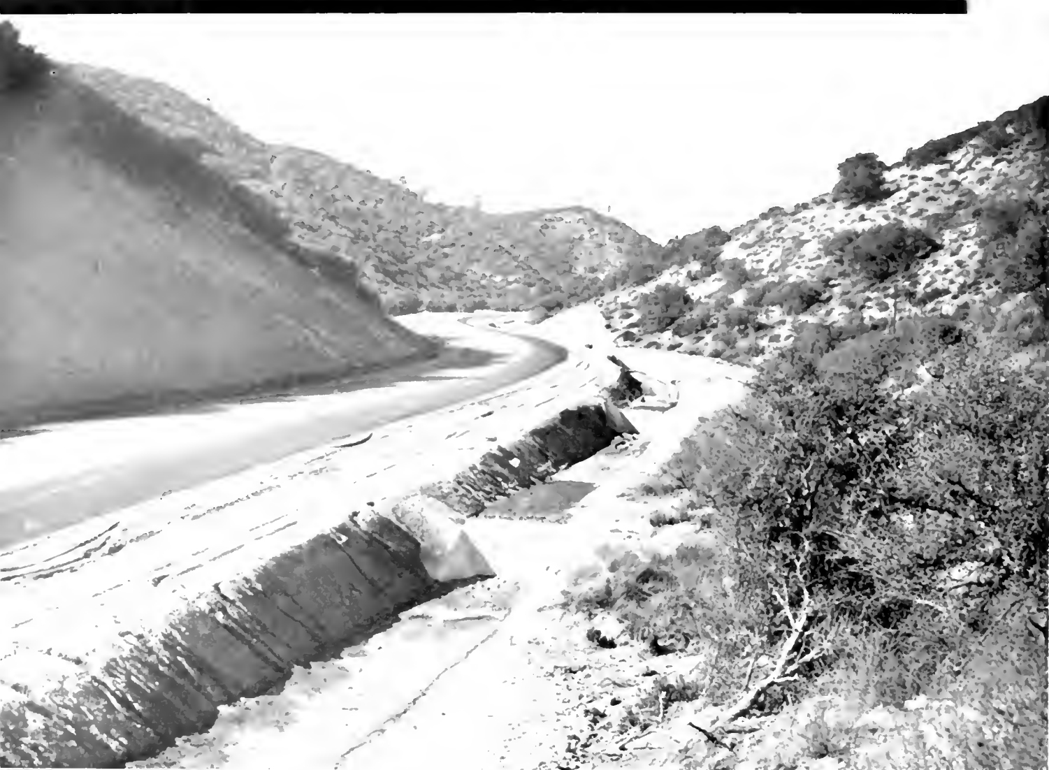
Section of Bradley-King City highway showing concrete check dams along creek channel to prevent excessive erosion in canyon section
